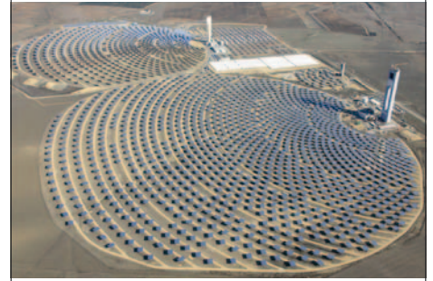
Figure 7: Commercial electricity production using solar tower concept – The 11 MW el PS10 plant (back) is in operation since 2007, and the 20 MW el PS20 plant (front) is in operation since 2009, both at Sanlúcar La Mayor near Seville, Spain.
